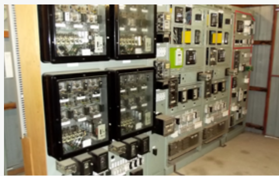
Figure 30. Fyshwick Zone Substation: Outdoor Wooden Pole Strung Busbars. Indoor 66kV Electromechanical Protection Relays
