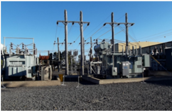
Figure 30. Fyshwick Zone Substation: Outdoor Wooden Pole Strung Busbars. Indoor 66kV Electromechanical Protection Relays
