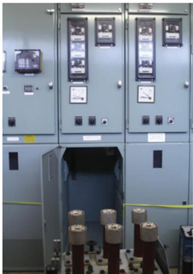
Figure 8. EXAMPLES OF VARIOUS HV APPARATUS WHICH IS TAPED AND/OR DANGER TAGGED TO CONTROL ACCESS TO VARIOUS PARTS OF THE APPARATUS
