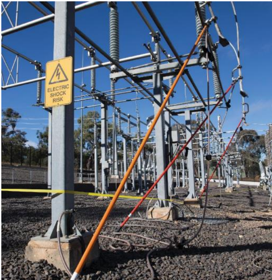
Figure 9. EXAMPLE OF OPERATIONAL EARTHS IN ZONE SUBSTATION
