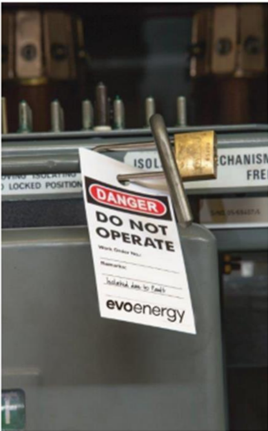
Figure 8. EXAMPLES OF VARIOUS HV APPARATUS WHICH IS TAPED AND/OR DANGER TAGGED TO CONTROL ACCESS TO VARIOUS PARTS OF THE APPARATUS
