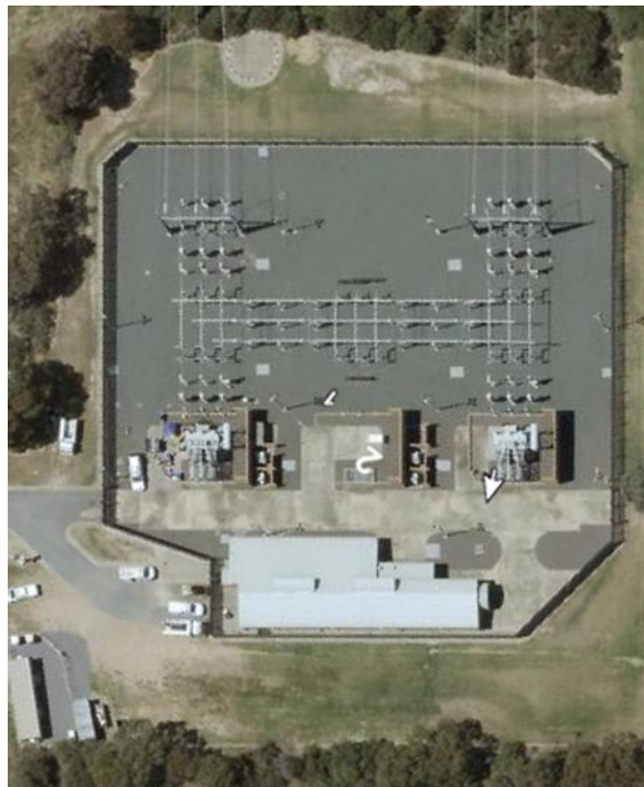
FIGURE 10: AERIAL VIEW OF GOLD CREEK ZONE SUBSTATION
