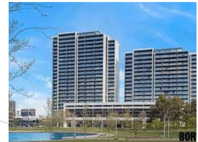
Images: examples of large complex buildings which will need to find and retrofit electric alternatives for existing gas uses such as domestic hot water.
