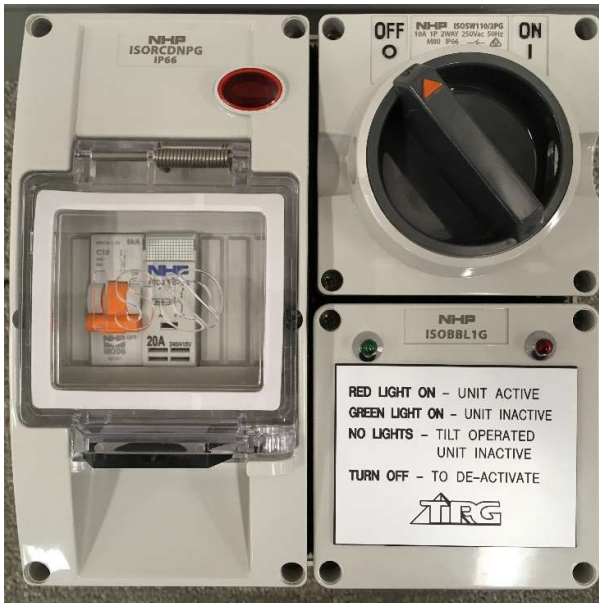
FIGURE 1. ISOLATION SWITCH ASSEMBLY
